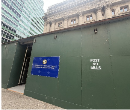
U.S. Bankruptcy Court Entrance One Bowling Green
