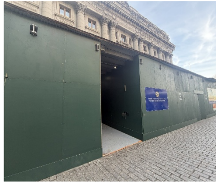
U.S. Bankruptcy Court Entrance One Bowling Green
